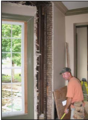
ABOVE LEFT: Kevin Duffey '79 removing the old plaster lath wall around the bay window. ABOVE RIGHT: The finished work around the living room bay window in the old wing. RIGHT: During and after the siding repair, painting, and new window installation on the south side of the old wing. Four new windows were installed in the living room, and the TV room received all new windows as well. BELOW: The stairs going from the Old Wing's landing to the second floor were repaired.
