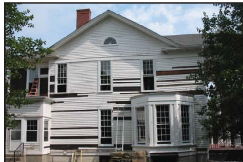
ABOVE LEFT: Kevin Duffey '79 removing the old plaster lath wall around the bay window. ABOVE RIGHT: The finished work around the living room bay window in the old wing. RIGHT: During and after the siding repair, painting, and new window installation on the south side of the old wing. Four new windows were installed in the living room, and the TV room received all new windows as well. BELOW: The stairs going from the Old Wing's landing to the second floor were repaired.
